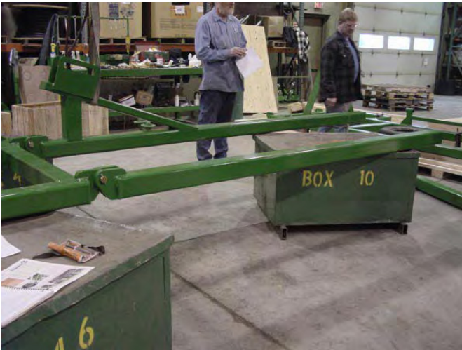
18. Left hand Wings leveled for further assembly.
